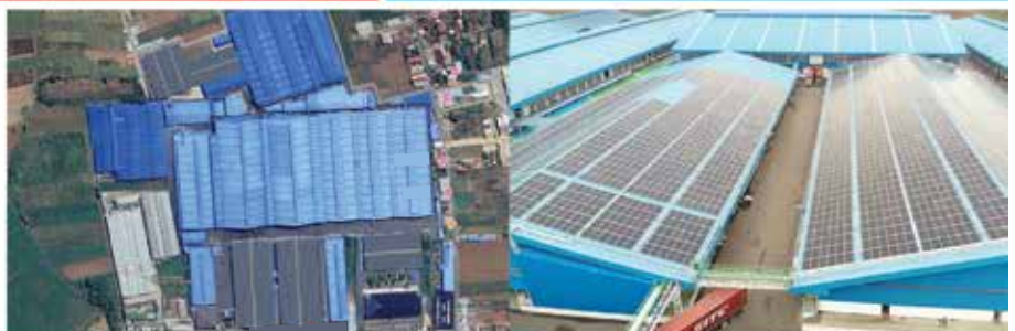
<PT. Hwa Seung Indonesia_Jepara_4.1MWp>
